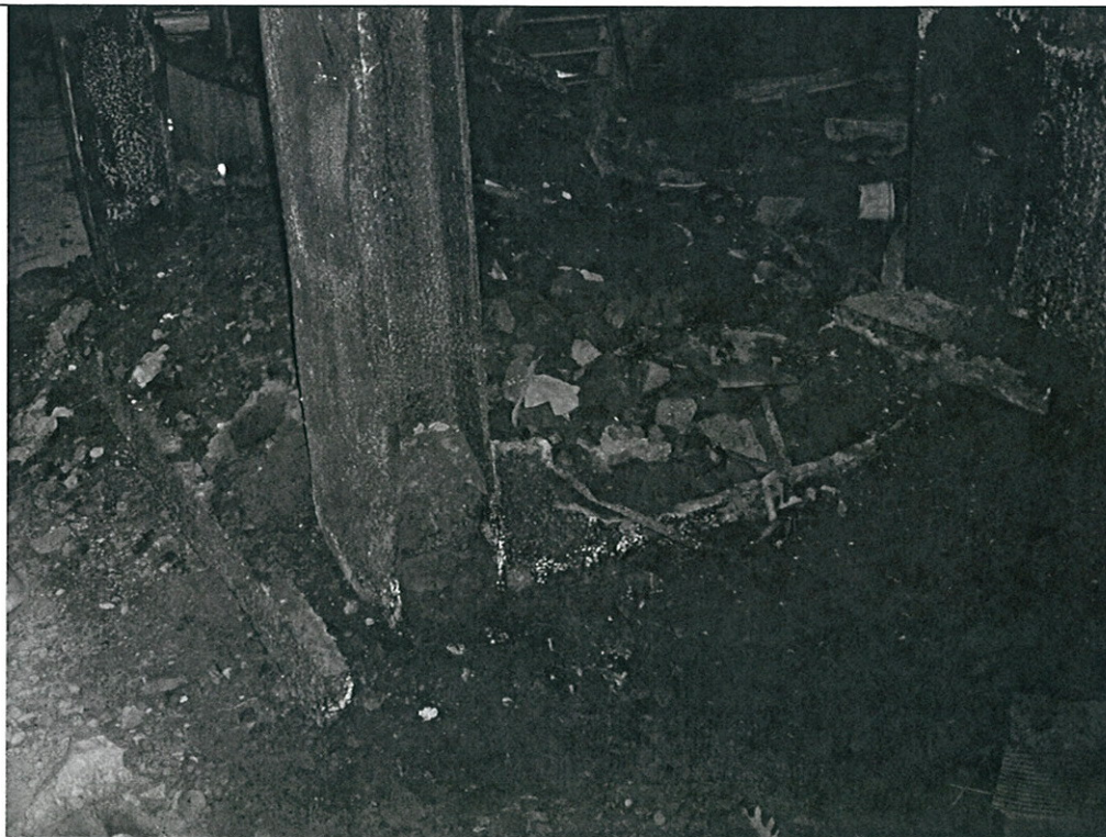
S-Special #9 – Black-stained soil around furnace foundation.
